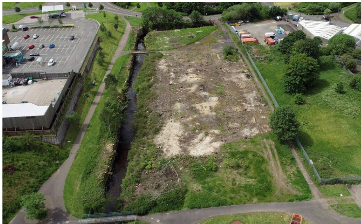
Figure 12: Levern Water during restoration works. Photo taken by AmcoGiffen Ltd. (contractor).
