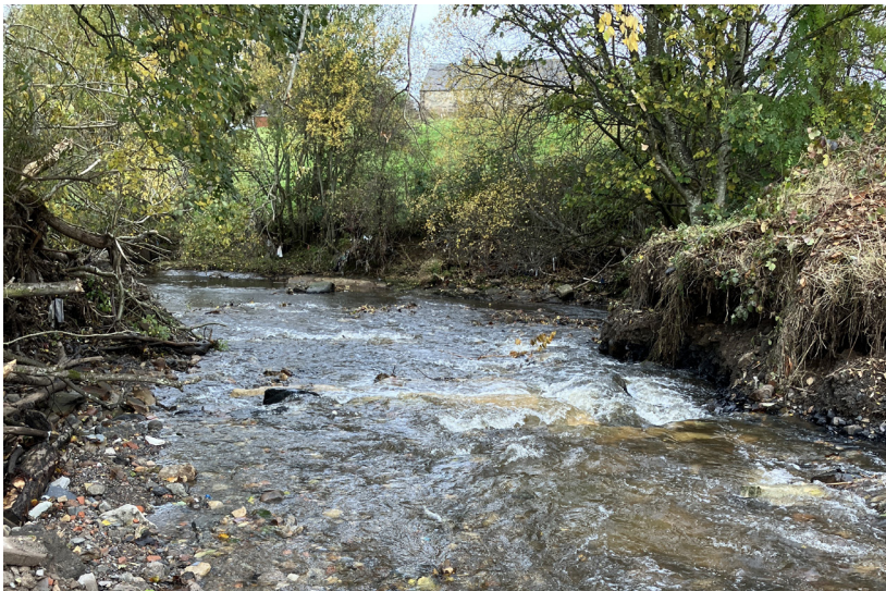
Figure 15: River Levern after removal of Crossmill Weir.
