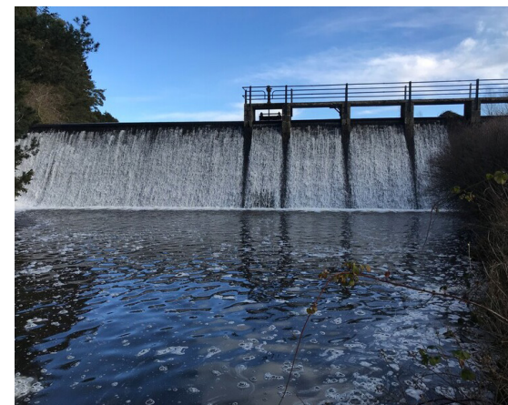
Figure 4: Garlogie Dam prior to removal.
