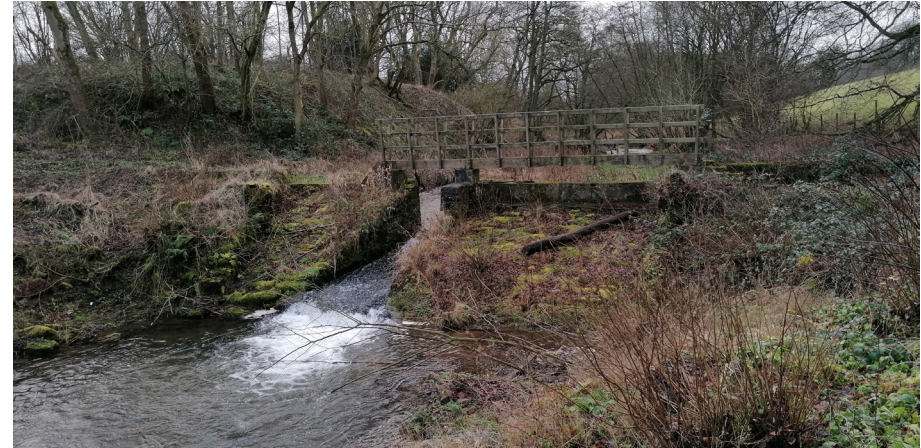
Before – Gateside Mills fish barrier in January 2022
